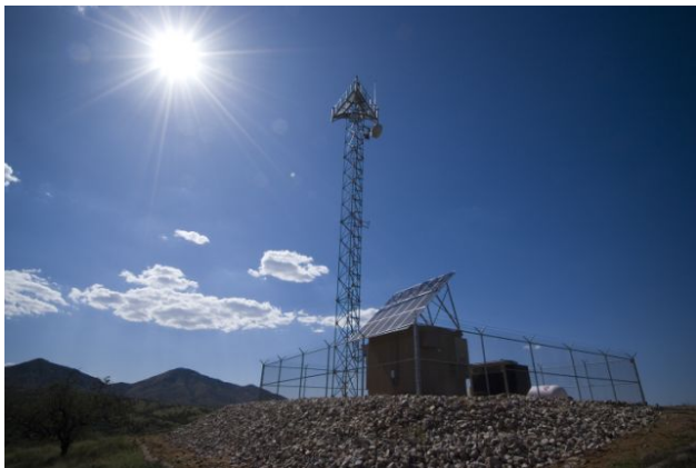
SBI net Block 1 Tower and support infrastructure in the Border Patrol's Tucson Sector.
